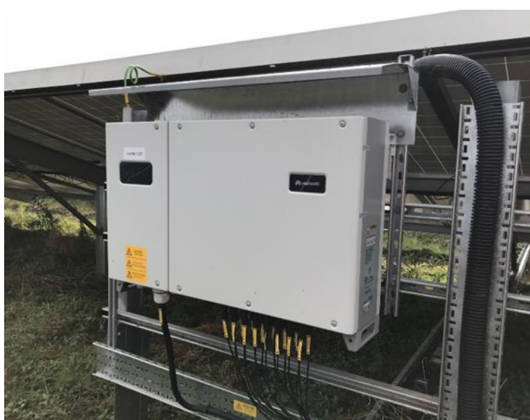
Figure 4-4 - Typical string inverter (image reproduced courtesy of Huawei)
